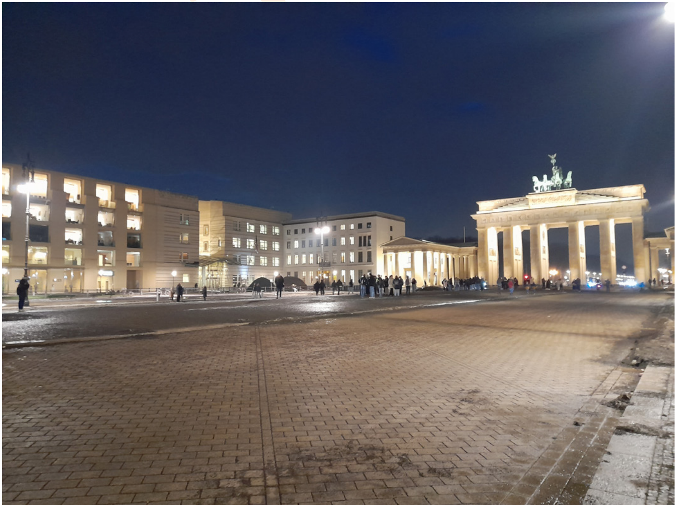
Fig. 2. Pariser Platz with the Brandenburg Gate and buildings reconstructed according to the principle of critical reconstruction. Source: Photograph by Boris Schwencke, 2026.
