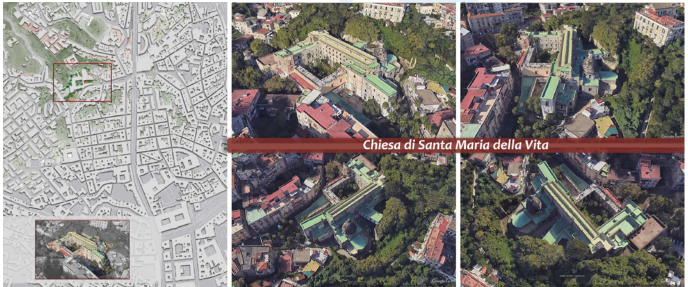
Fig. 1. Location and aerial views of the Church of Santa Maria della Vita within the urban context of the Sanità district, Naples, highlighting the relationship between the church, the former monastic complex, and the surrounding topography (prepared by R. Iaderosa).
