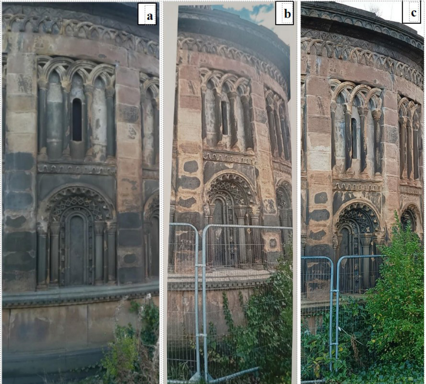
FIG. 5: Comparison of the decay progression in the North-West Niche (NW4) in 2017 (a), 2023 (b) and 2025 (c).
