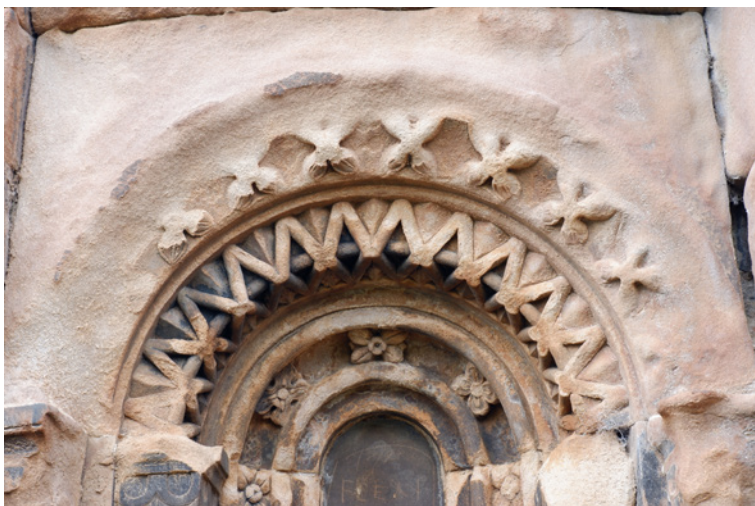
Figure 4: South-east niche showing the loss of carved detail (picture from 2020).
